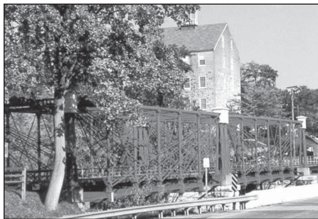
Figure 3.3. The color and historical industrial design character of the Bollman Bridge is the inspiration for street furniture along Route 1.
