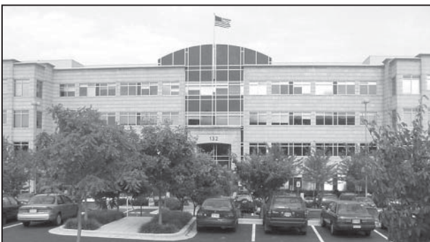
Figure 5.2. Although one-story flex space and light industrial buildings will continue in the corridor, multistory office buildings are encouraged in the corridor zoning districts.
