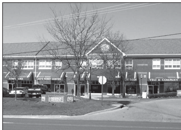
Figure 5.13. Locating signs on canopies or on special wall-mounted sign panels provides a consistent and attractive appearance.
