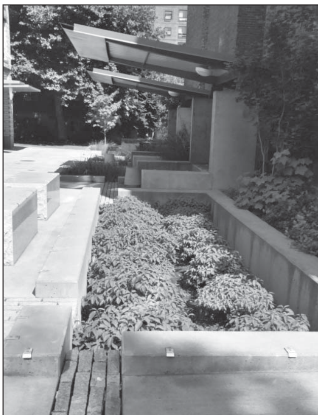
Figure 4.20. Bioretention areas can be designed attractively to suit urban stormwater management conditions.
