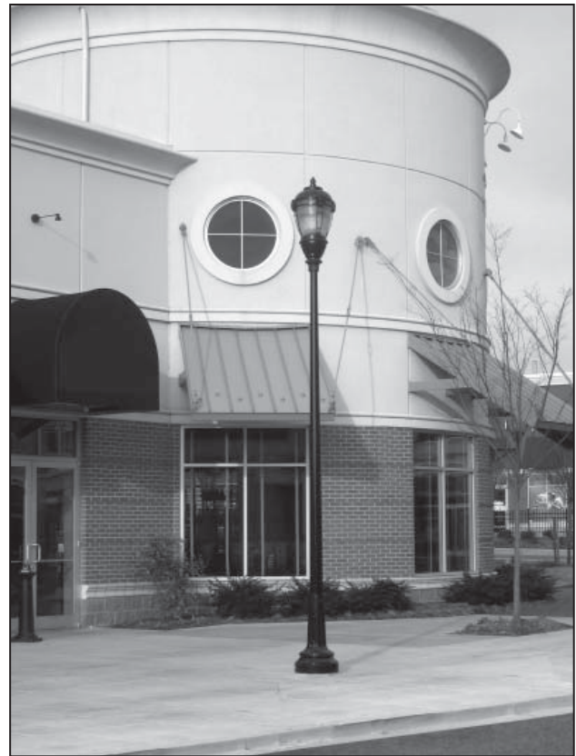
Figure 3.21. The ornamental pedestrian street light selected for the Route 1 corridor is an acorn full cut-off fixture atop a 12-foot tall black finish pole with fluted shroud base. The selected light is subject to change.
