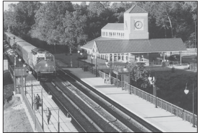
Figure 1.5. Transit oriented development means convenient access to train and bus routes with attractive train stations and bus shelters.
