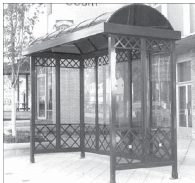
Figure 3.17. The recommended bus shelter for the Route 1 corridor is Slimline, 5-foot by 10-foot, black or red powder-coated metal, manufactured by Brasco International, Inc., or equal by another manufacturer.
