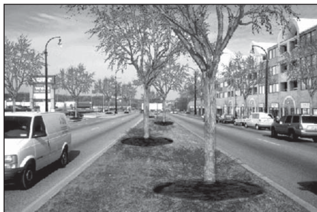
Figure 3.4. Where space allows, a landscaped median can control traffic movements, increase pedestrian safety and make a more attractive roadway.
