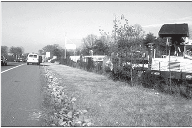
Figure 4.15. Exposed storage areas along Route 1 enclosed with chain link fence are unsightly.
